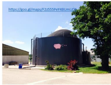
France: 10.000 m 3 pig slurry = 27 TPD = 50kW with bert 600 m 3 = 430.000 kW/h el.per year
