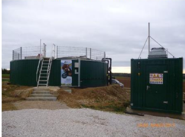
Typical bert project in concrete Digester in concrete and technical container
